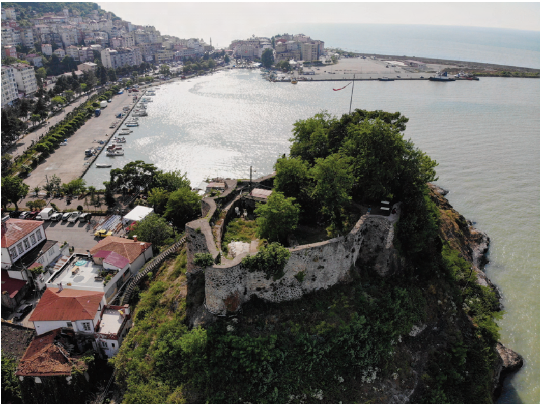
Plate 54. Tripolis (Tirebolu). View of the fortification. ( Source: Karadeniz Kültür Envanteri)
